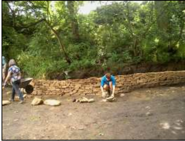
Dry stonewall being restored by Mick and volunteers
